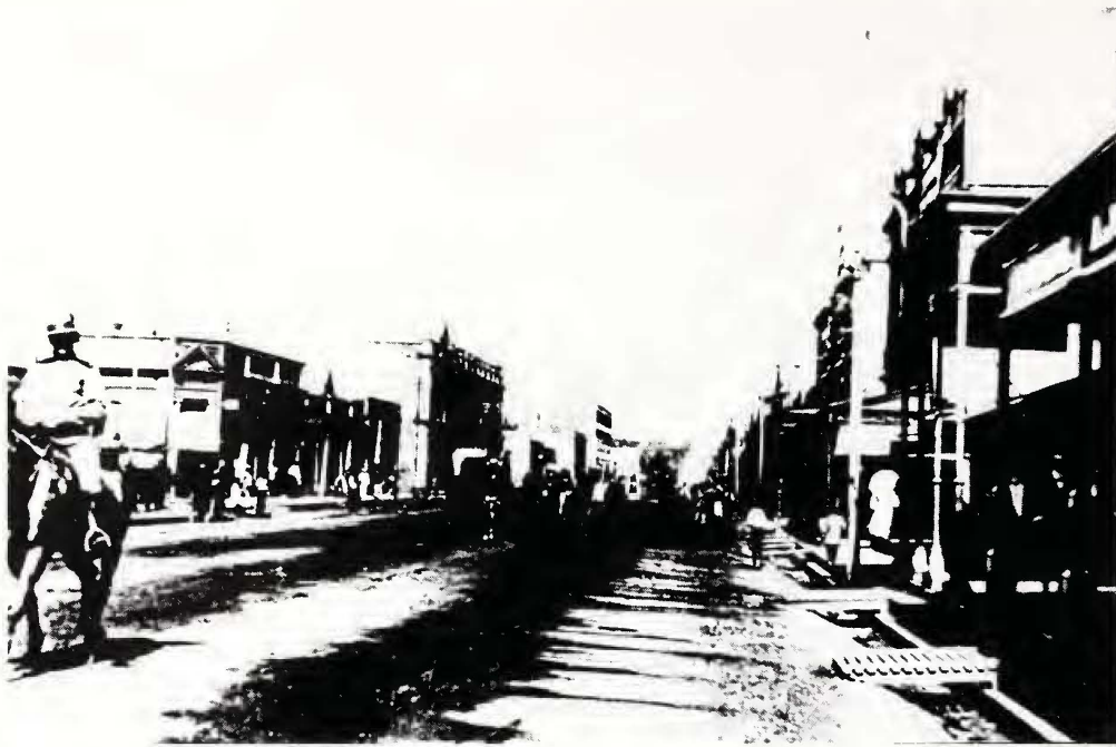
Fig. 7. A photograph of Church Street East in 1904. The function of the shallow furrow on the southern side (on the right) next to the kerbstone, was to drain storm water to inlets in the sidewalk. The photo indicates that the furrow under investigation was still used in 1904 and that it was a stormwater ditch (Dunston 1975:141).
