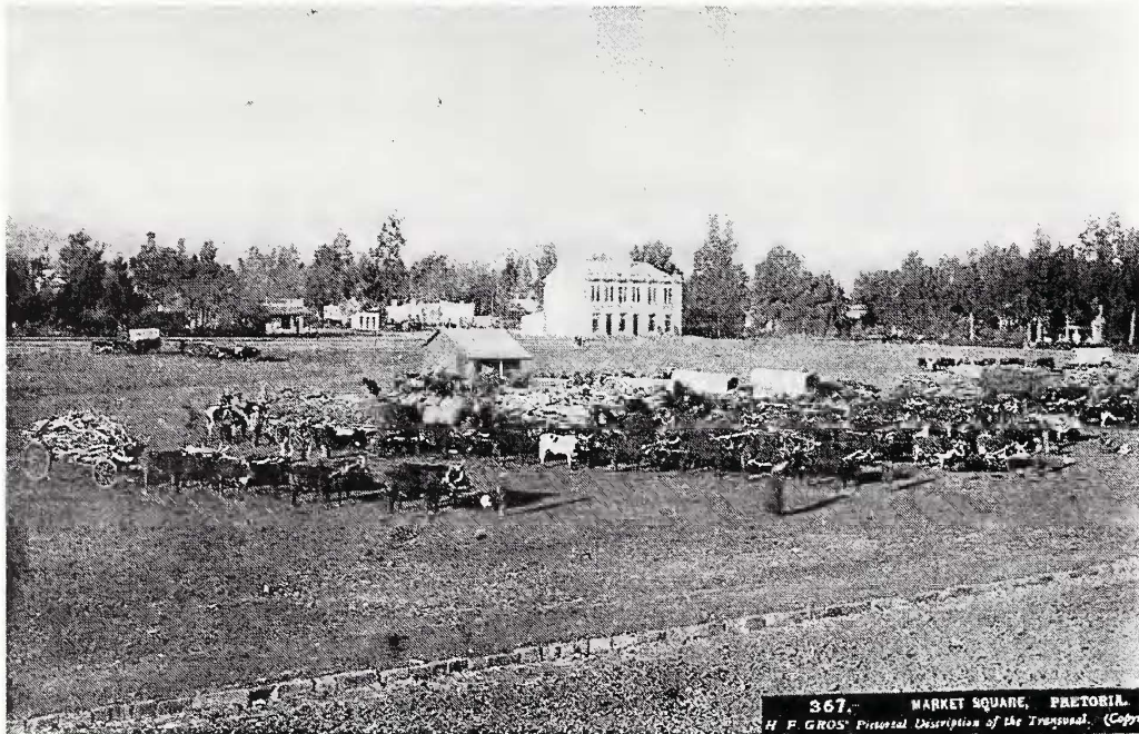
Fig. 8. This photograph clearly shows a water inlet in the kerbstone (bottom left) at the investigated area (Gros n.d.:367).
